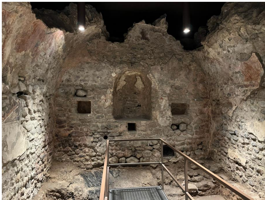
Fig. 5. St. Stephan Crypt – Underground Church in Coira
